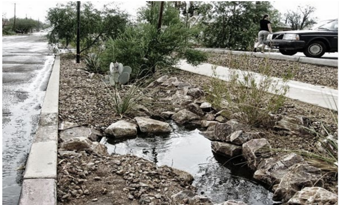
Curb cut and bioretention swale on Cherry Avenue, Tucson by Watershed Management Group
