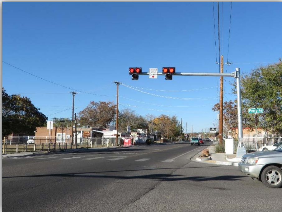
Figure 5-21: Pedestrian Hybrid Beacon in Bernalillo County
