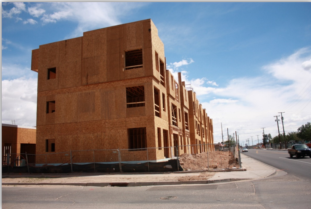
Figure 2-9: New Housing Construction in the AMPA
