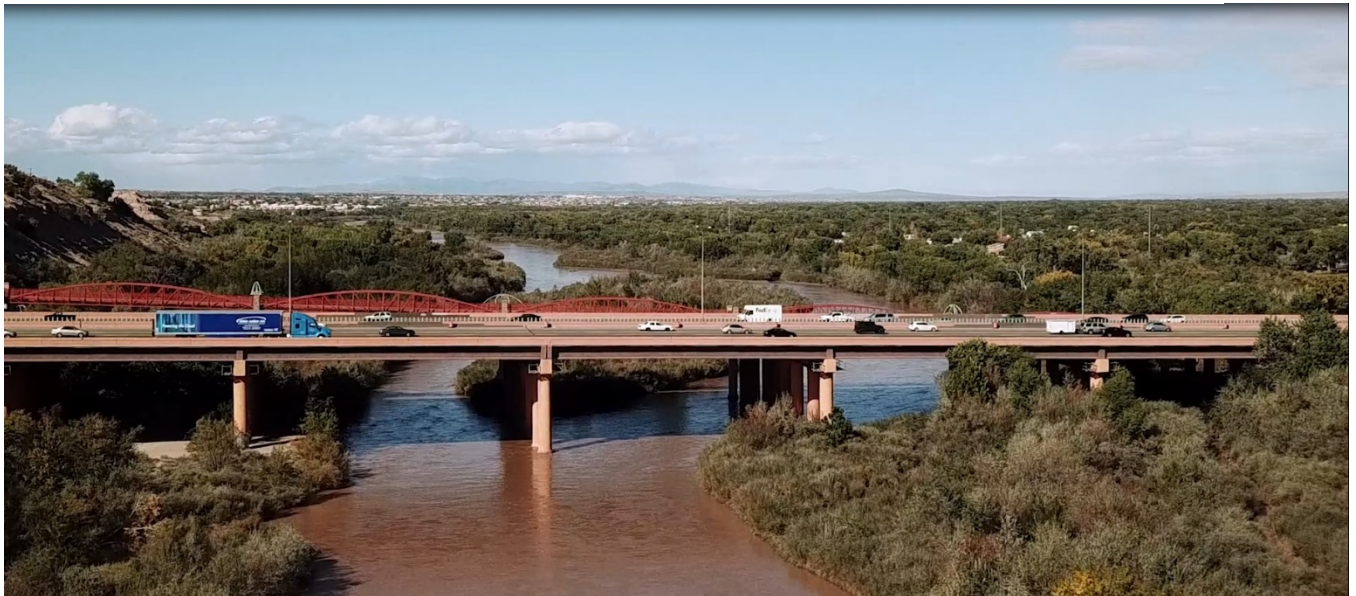
Figure 4-9: River Crossing in the AMPA
