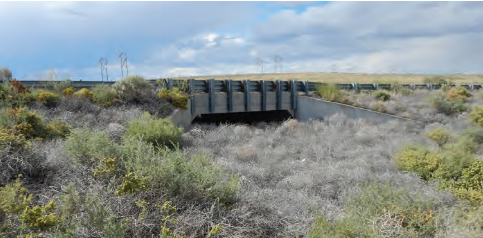
Atrisco Vista Boulevard Crossing at the North Fork Boca Negra Arroyo.
