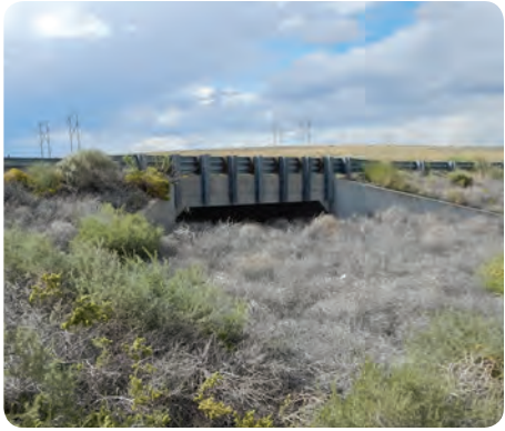
Existing drainage facility.
