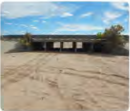
Existing drainage facility.
