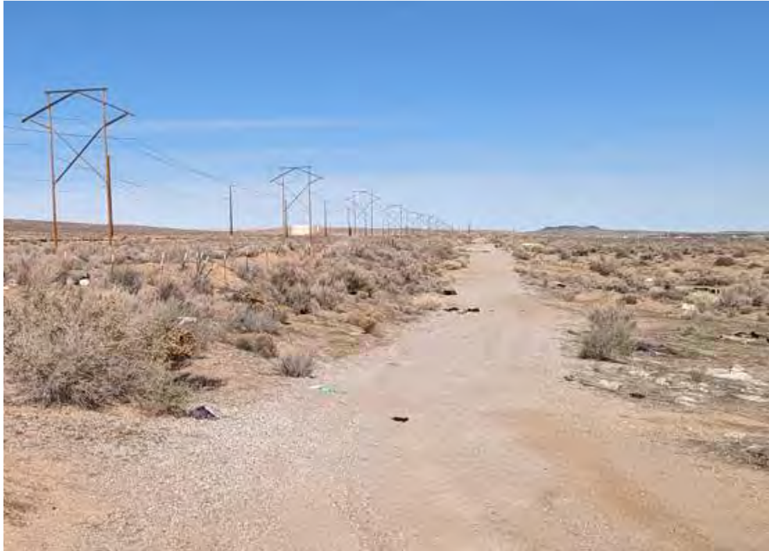
Figure 2: 118 th Existing Conditions
