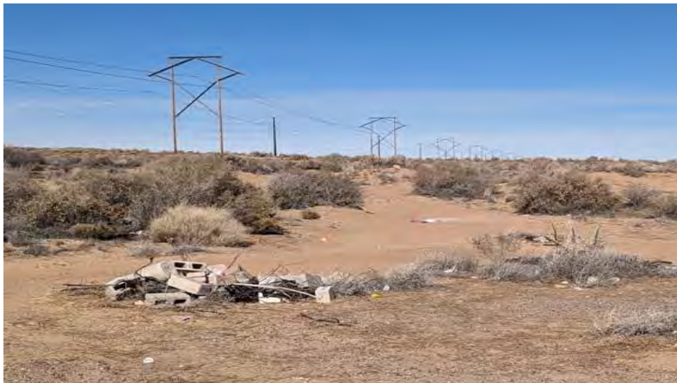
Figure 3: PNM Transmission Lines along 118 th Street
