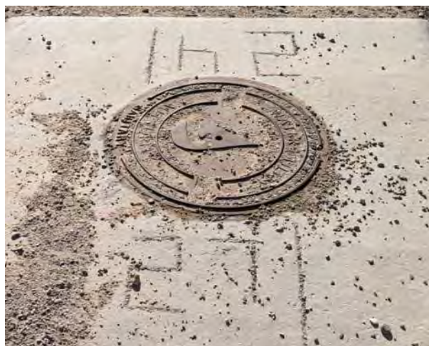
Figure 4: Existing Sewer Manhole
