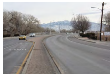
View of Rio Grande bridge (east)
