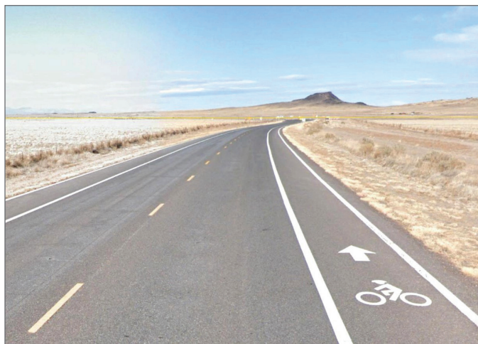
Eight-foot shoulders striped as bicycle lanes.
