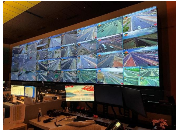
New Mexico DOT Regional Traffic Management Center (RTMC) located in Albuquerque, NM.
