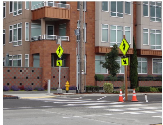
Solar-powered RRFs can be mounted to metal or wooden signposts at crossings.
