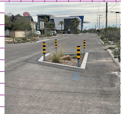
A chicane in Tucson, Arizona calms traffic and also serves as green stormwater infrastructure.
