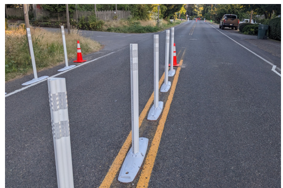
Flexible delineator posts installed along centerlines and edge lines encourage slower speeds.
