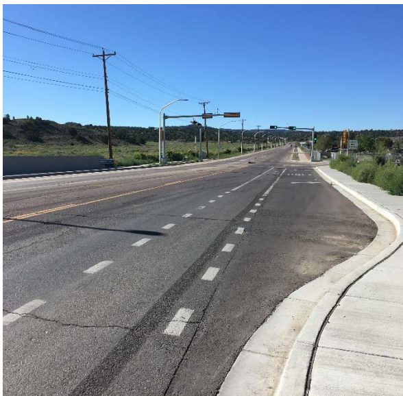
In 2017, NMDOT installed bike lanes along Boardman Drive (NM 564) in Gallup, NM as part of a road diet that converted the roadway from a four to three-lane cross-section.
