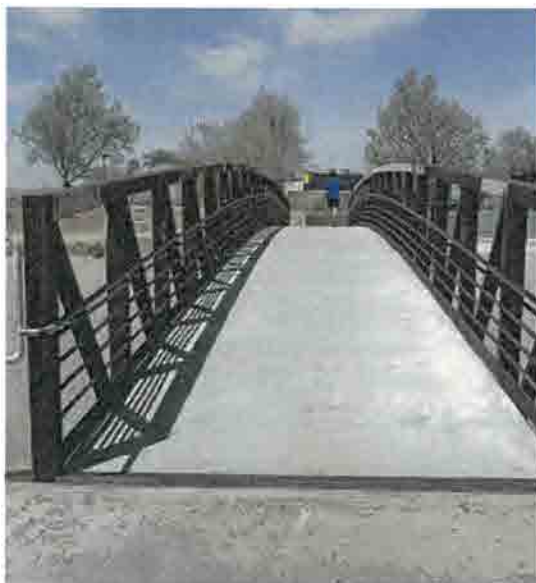
North Diversion Channel Bridge, ABQ
