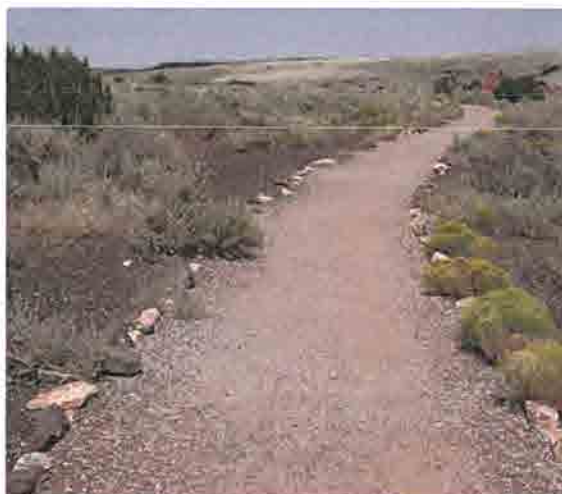
Compacted Crusher Fines Surfacing
