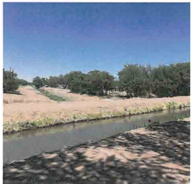
FIGURE 14. NO CROSSING OVER ARENAL MAIN CANAL
