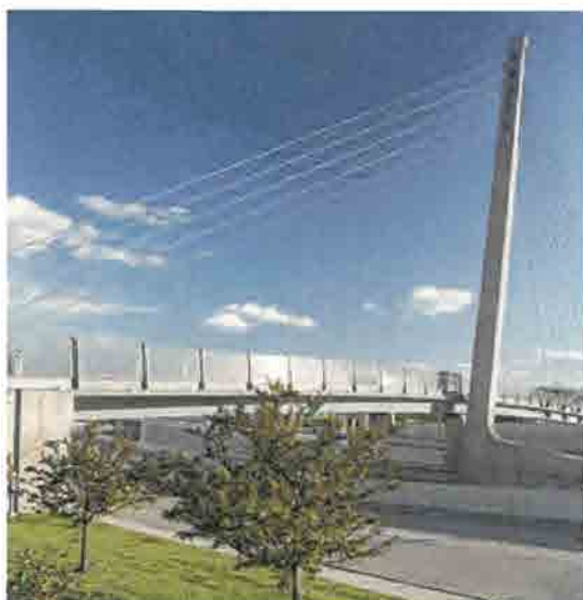
Bagley Pedestrian Bridge, Detroit
