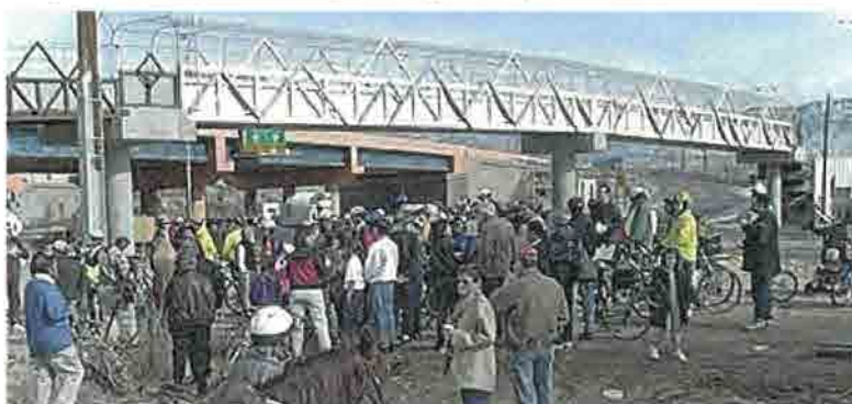
2nd Street Bridge, Albuquerque
