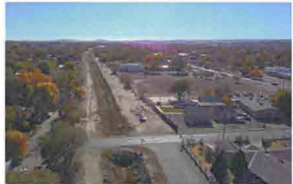
Looking South at San Ignacio Road Crossing
