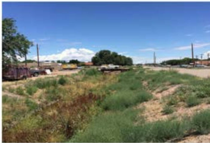
Looking north along the Alameda Drain adjacent to 2 nd Street.
