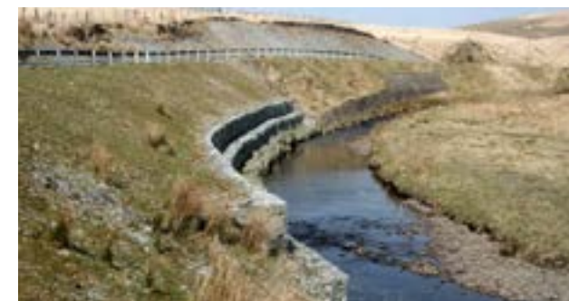
▲ GABIONS STABILIZING RIVER BANKS
