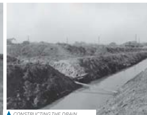
▲ CONSTRUCTING THE DRAIN
