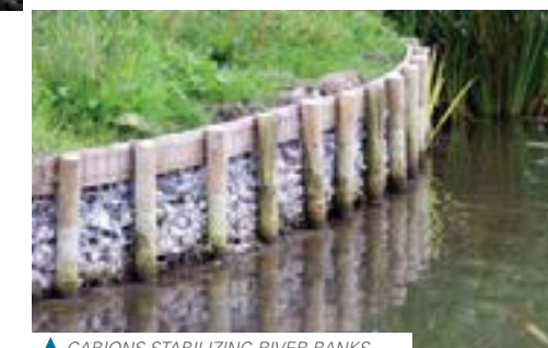
▲ GABIONS STABILIZING RIVER BANKS
