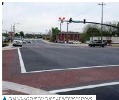
▲ CHANGING THE TEXTURE AT INTERSECTIONS
