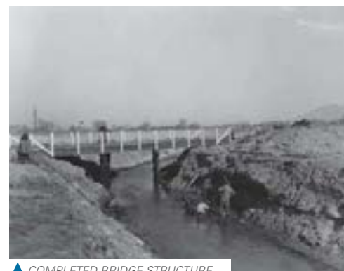
▲ COMPLETED BRIDGE STRUCTURE
