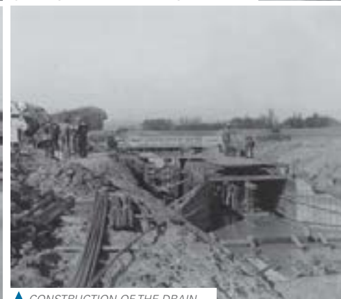
▲ CONSTRUCTION OF THE DRAIN
