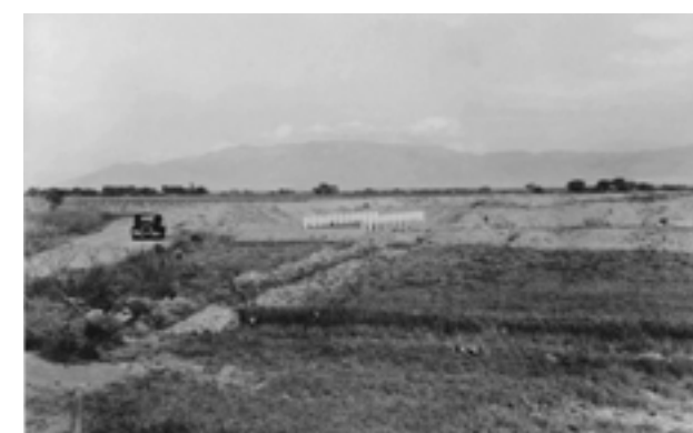
View showing new highway bridge over Alameda Interior Drain where the course of the Drain makes it necessary to divert the highway
