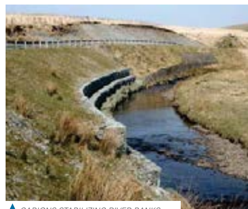
▲ GABIONS STABILIZING RIVER BANKS
