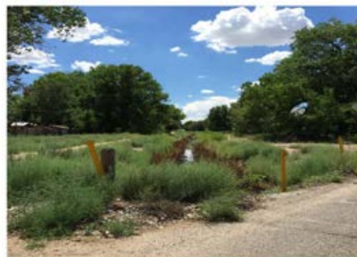
Alameda Drain and adjacent pathways in the northern portion of the project corridor between the AMAFCA North Diversion Channel and 2 nd Street.
