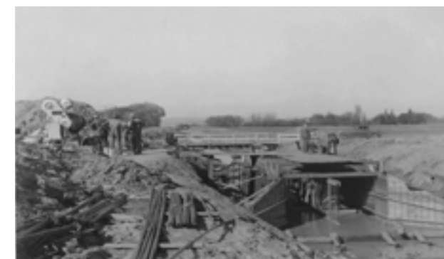
View showing construction of concrete culvert on Highway 66 at the point of the Alameda Interior Drain crossing.
