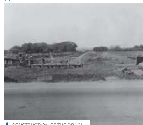
▲ CONSTRUCTION OF THE DRAIN
