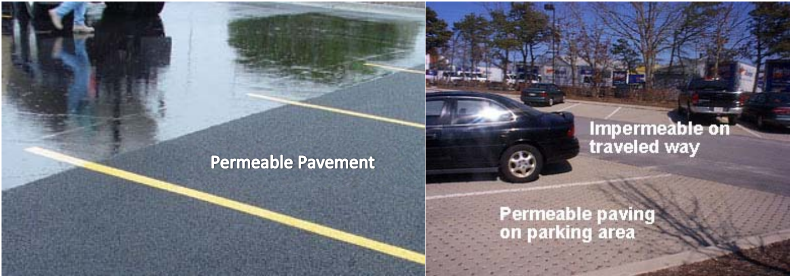
Examples of Permeable Paving for the parking area and conventional pavement on the driving/travel lanes
