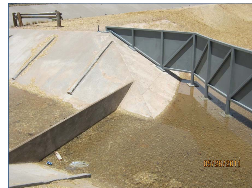
Example of a Baffle/Weir Wall Water Quality Structure used for AMAFCA's Grantline Water
