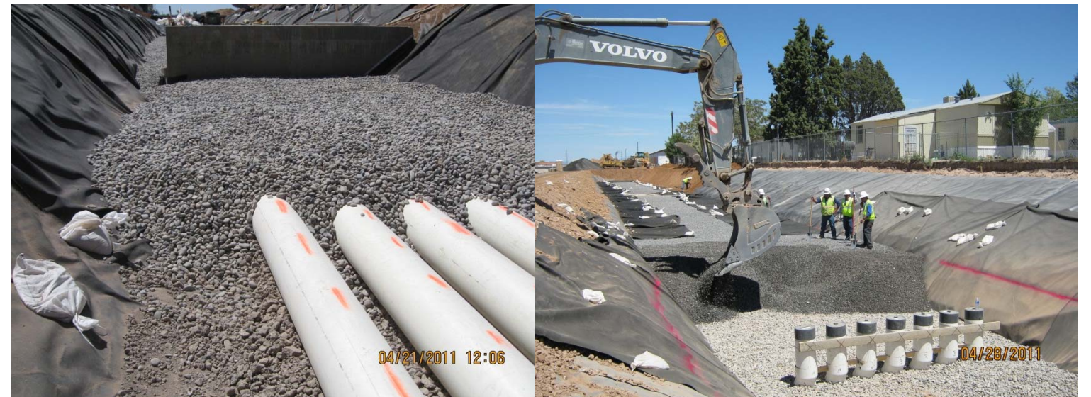
Media Filter Settling Basin – AMAFCA's Candelaria Water Quality BMP during construction
