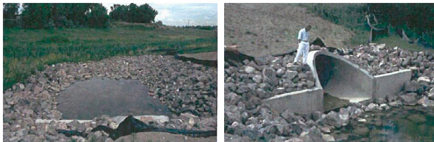
FIGURE 6.10.22 Upstream and Downstream Views of a Low Tailwater Basin in Douglas County
