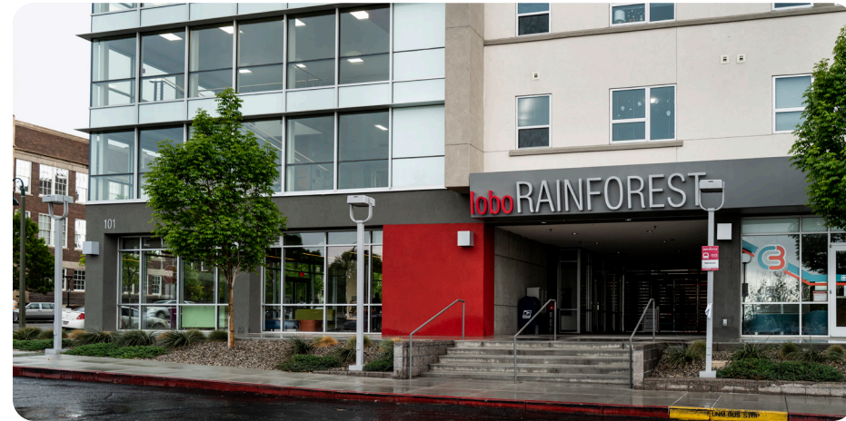
Lobo Rainforest Building (City of Albuquerque)
