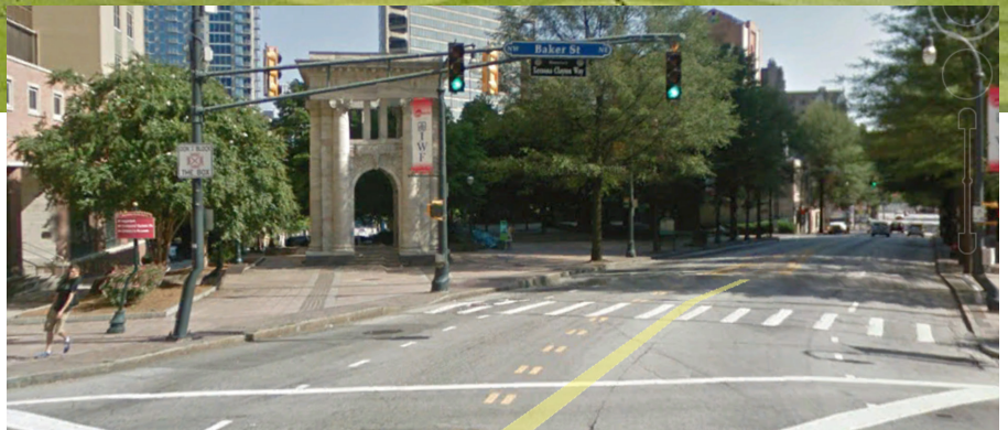
■ Peachtree Street, Atlanta, GA Pedestrian Esplanade and arch where traffic used to flow on Peachtree Street in Atlanta, GA (Source Google)
